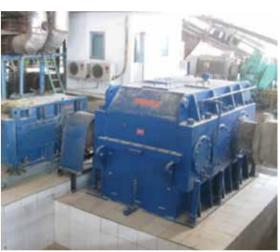
Based on David Brown's renowned range of industrial reducers, applications specific drives for the sugar industry can be rapidly configured from standard designs and components. High torque direct mill drive units can be provided fitted with input and output couplings and can be fitted with integral reversing drives and lubrication systems.
